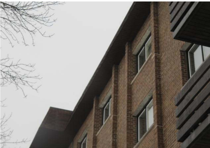
Overview of soffits at mansard roofs.
