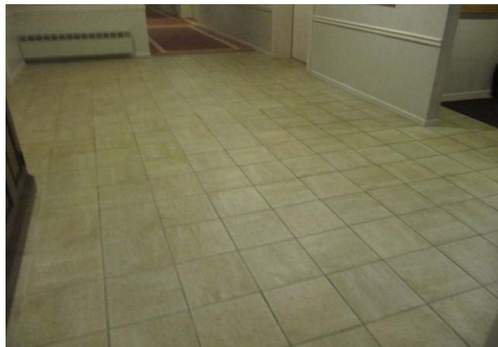
Overview of tile floor at lobby.
