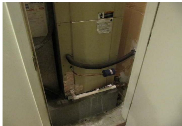
BDP Company brand fan coil unit.
