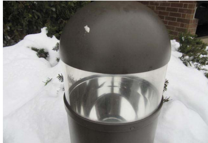
Bollard light fixture near building entrance.
