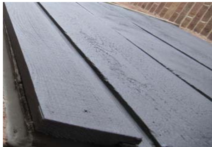
Wood siding panels are in good overall condition.
