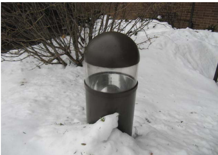
Typical style and condition at bollard light fixture.
