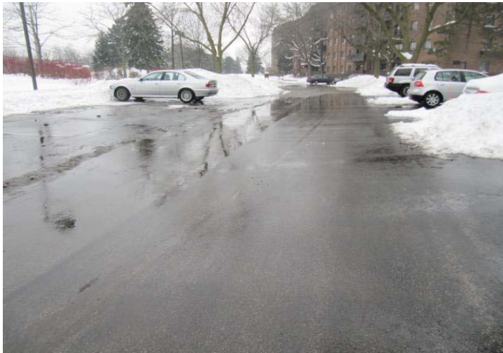
Overview of asphalt pavement at parking lot.
