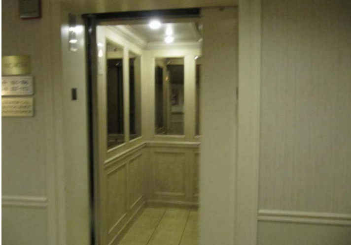
Overview of elevator cab interior.
