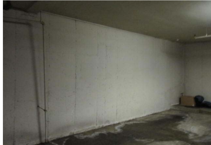
Overview of painted wall at parking garage.
