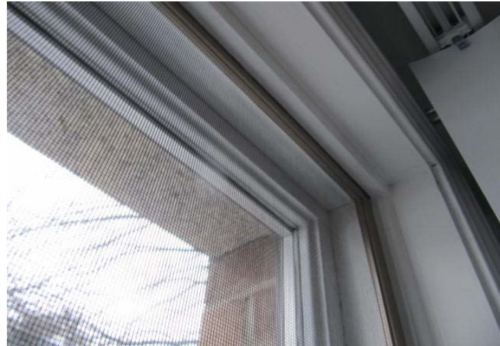
Interior view of wood casing at common window.
