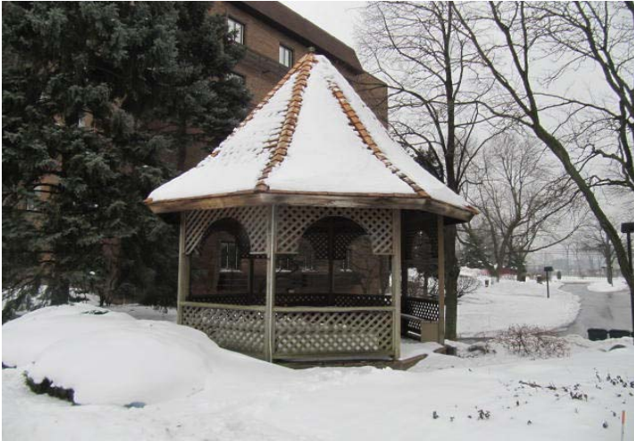
Overview of wood gazebo.
