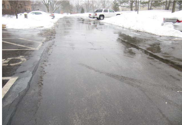
Asphalt pavement at drive aisle.
