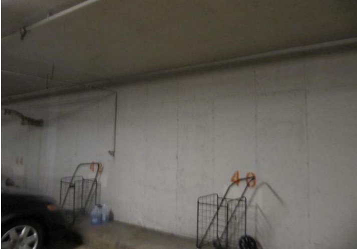
Overview of painted wall at parking garage.
