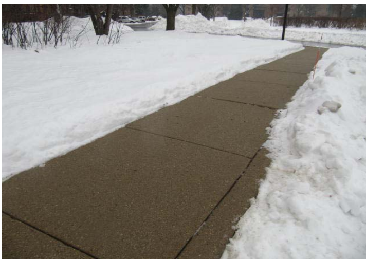
Area of sidewalk in good overall condition.
