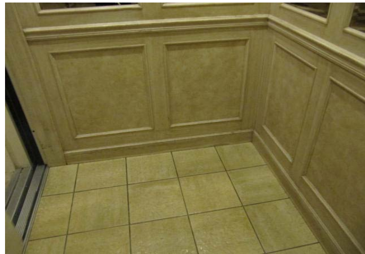
Tiled floor and wood wall panels at elevator cab interior.
