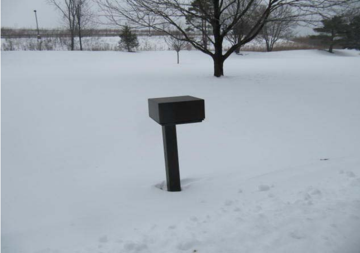
Typical light fixture along fire lane.
