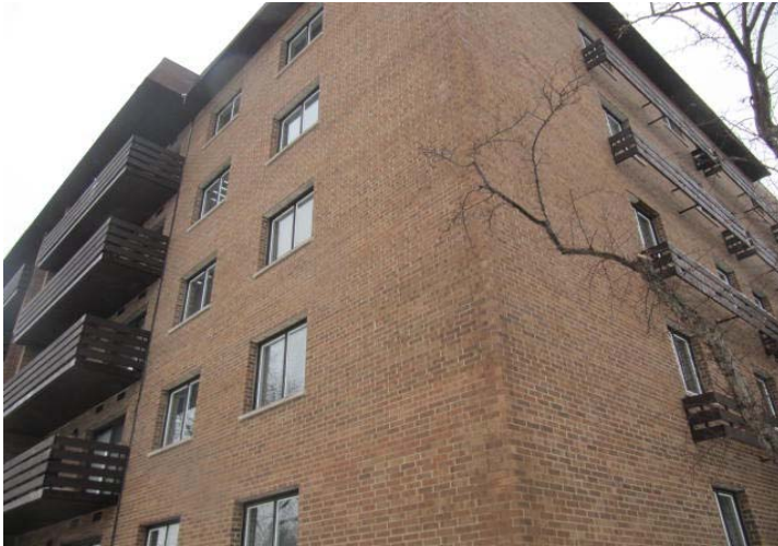
Overview of masonry façade.
