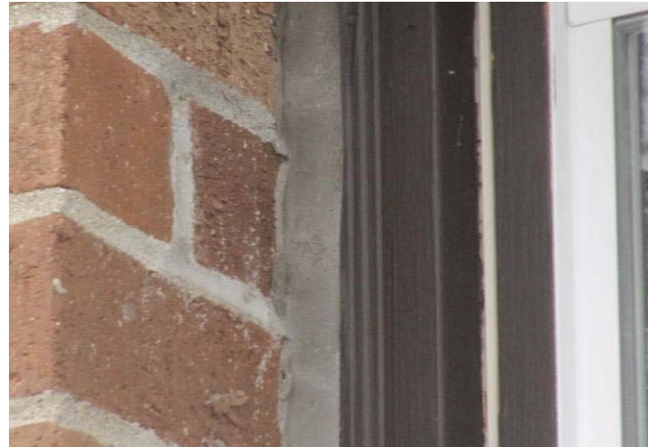
Sealant at unit window, in good overall condition.
