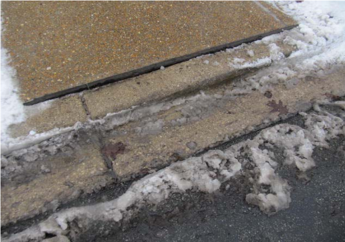
Concrete curb and gutter at perimeter of parking lot.
