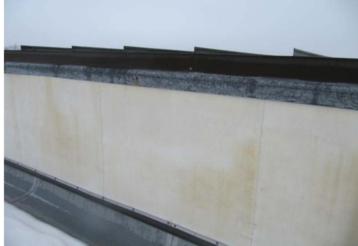
Overview of parapet wall at building roof.
