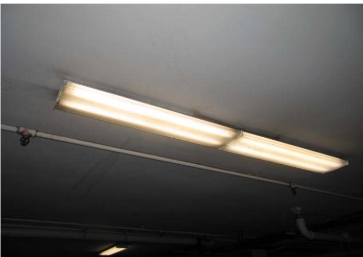
(2) light fixtures back-to-back
