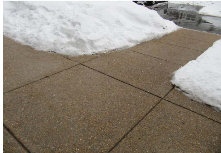
Concrete sidewalk, with exposed aggregate finish.
