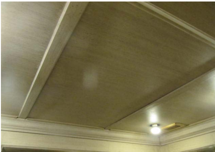
Wood ceiling at elevator cab interior.
