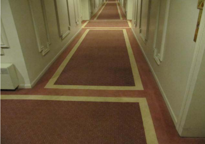
Overview of carpet flooring at hallway area.
