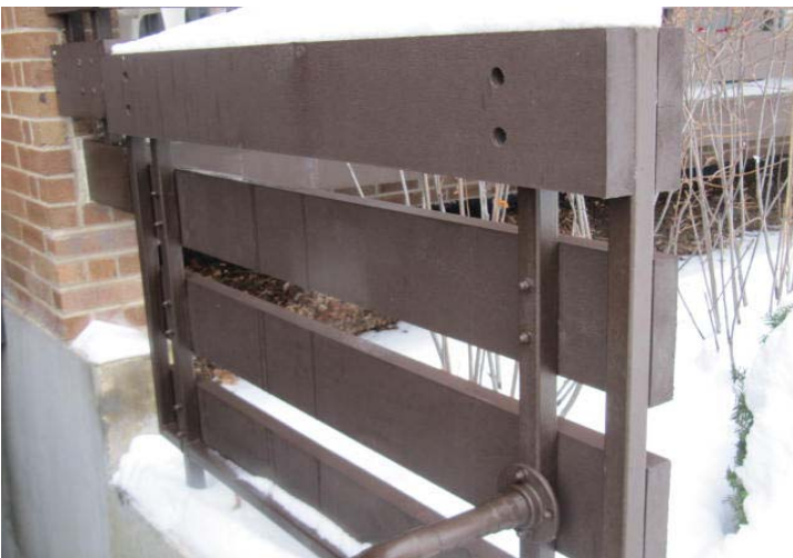
Railings at private stairwell door.
