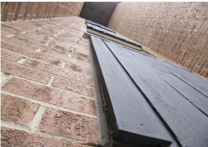
Sealant between masonry façade and wood siding.
