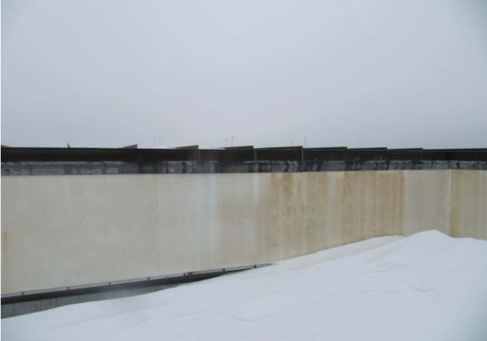
Overview of parapet wall at building roof.
