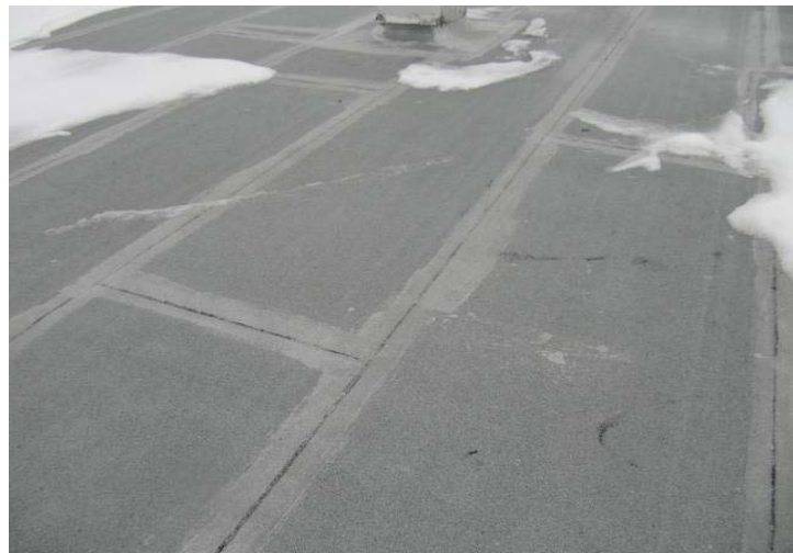
Building roof, replaced in 2006.
