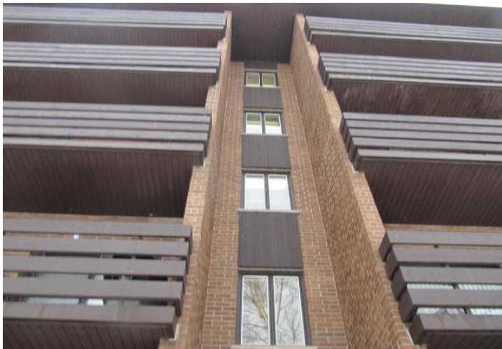
Overview of painted wood siding and railings.
