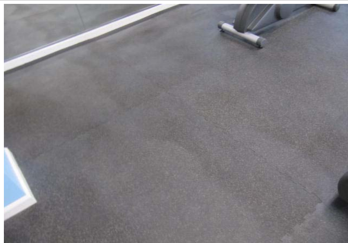
Rubber sports flooring, in very good condition.
