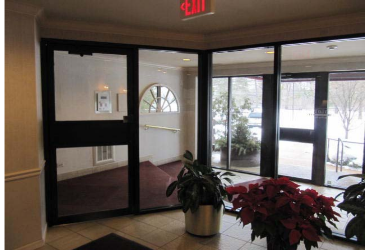
Interior view of glazing and entry doors.
