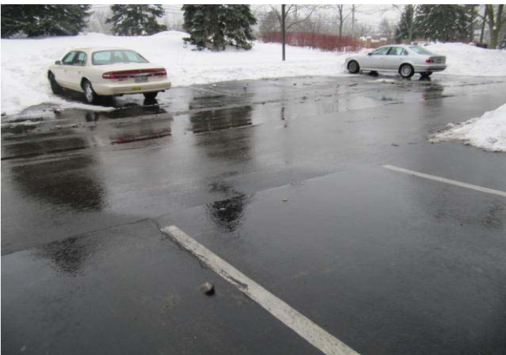
Overview of asphalt pavement at parking lot.
