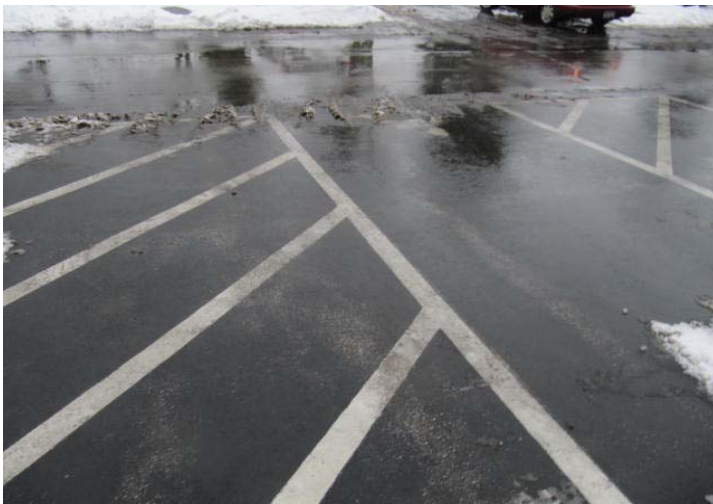
Clear marking at handicap parking stall.
