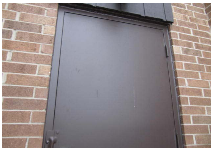
Paint finishes at exterior surface of solid door.
