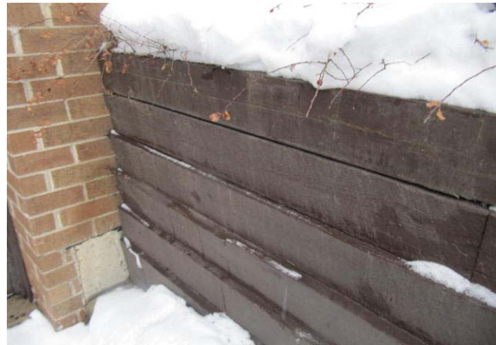
Timber retaining wall near garage entrance.
