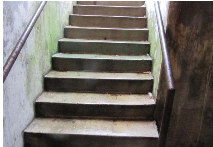
Concrete formed stairs, viewed from garage level.
