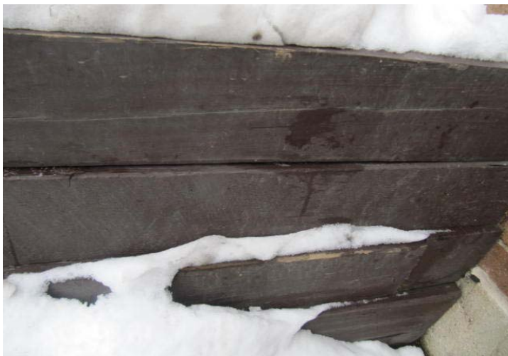
Typical timber retaining wall, with paint finishes.
