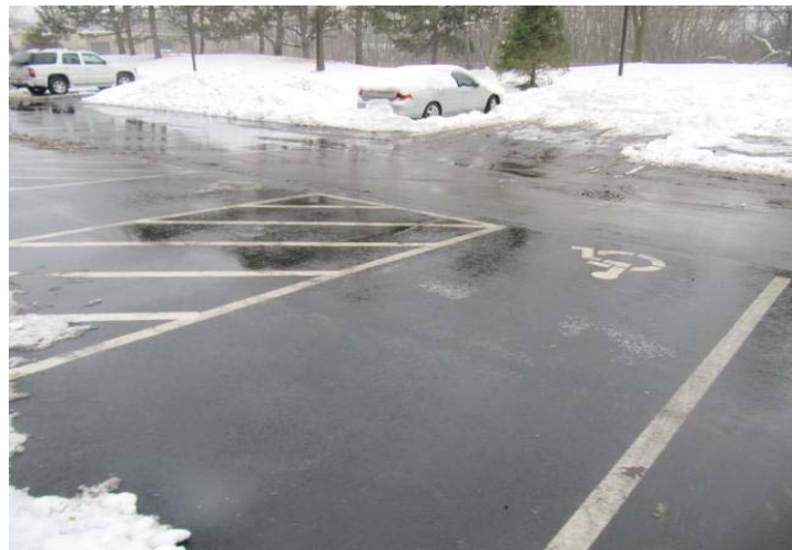
Asphalt pavement at parking bays.
