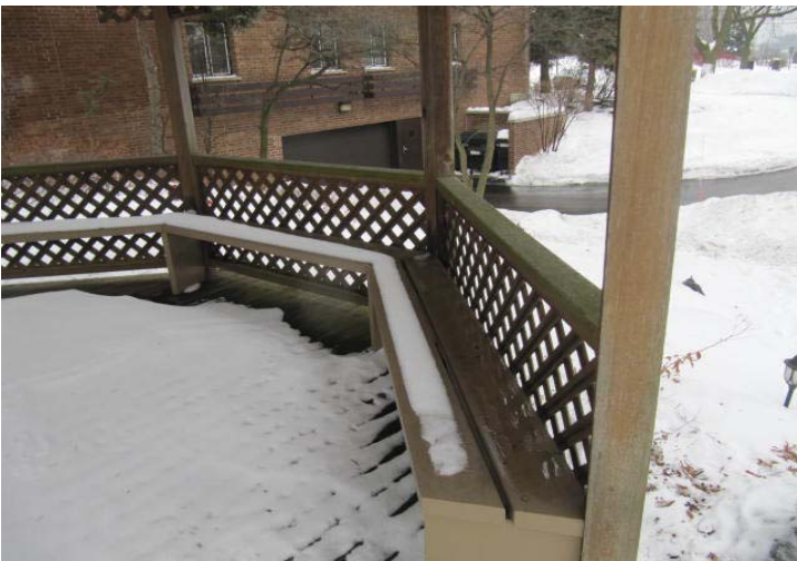
Railings and benches at gazebo.
