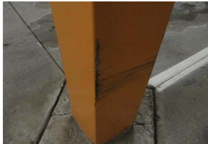
Markings at structural concrete column.
