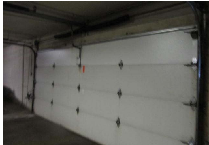
Insulated, sectional door with springs, coils, and track.
