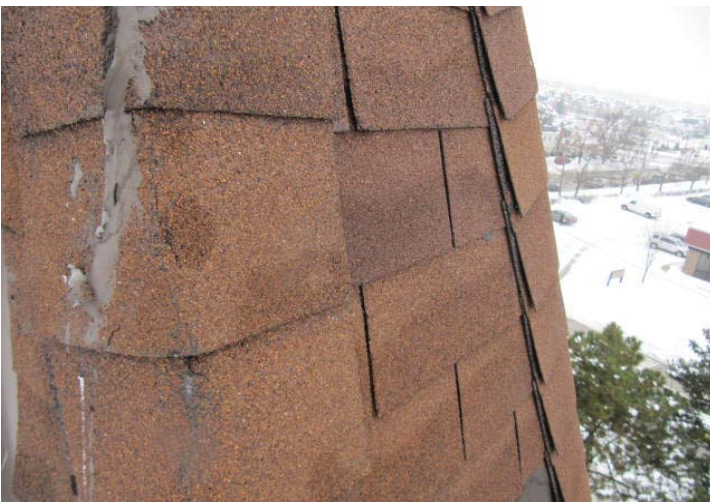
Asphalt shingles, in fair condition.
