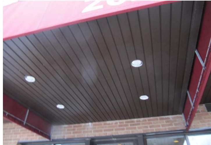
Soffit at underside of entry canopy.
