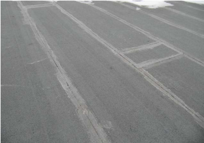
Overview of flat modified bitumen roof.
