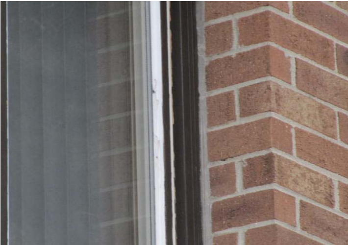
Sealant at perimeter of unit window.
