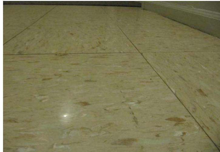
Vinyl tile at lower level garage elevator lobby.
