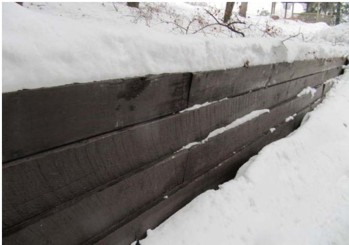
Timber retaining wall along entry drive to garage.
