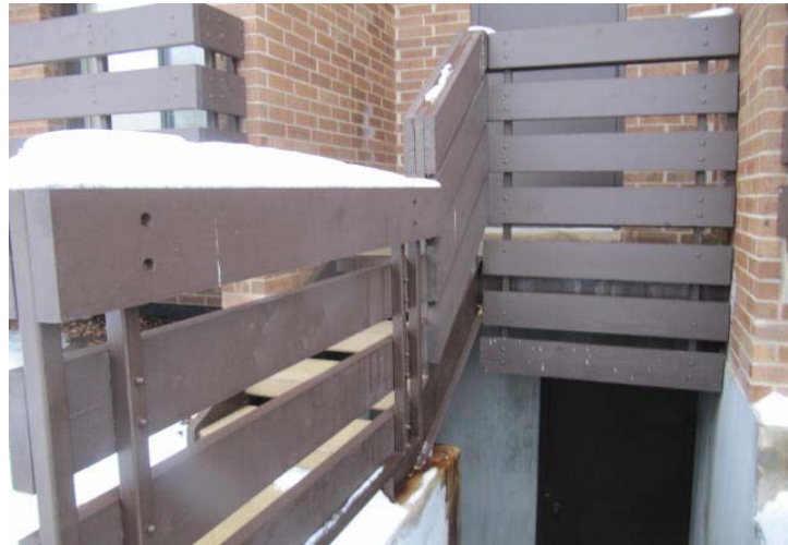
Railings at private stairwell door.
