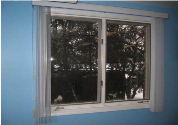
Interior view of window at exercise room.
