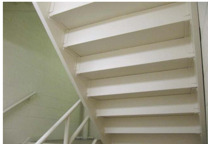
Painted underside of metal stair structure.
