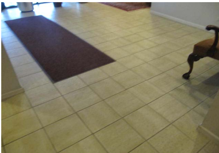
Overview of tile floor at lobby.
