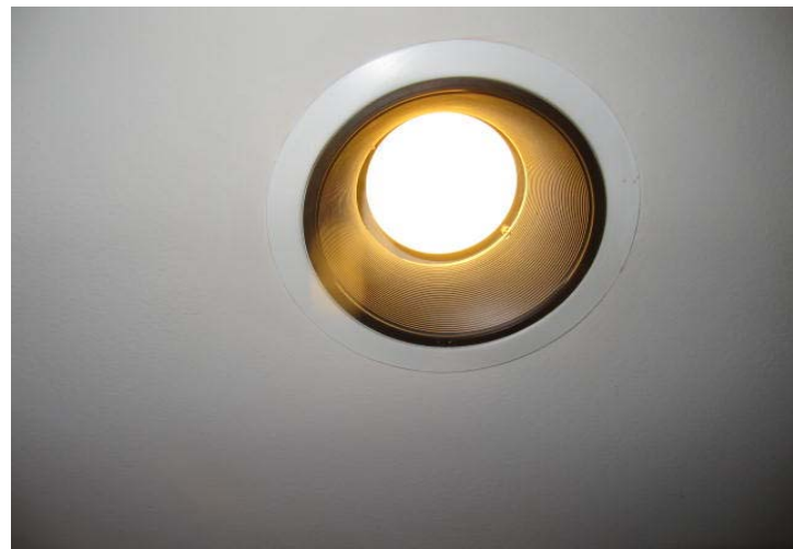
Typical recessed can light.
