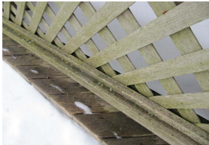
Lattice panel and wood floor boards.
