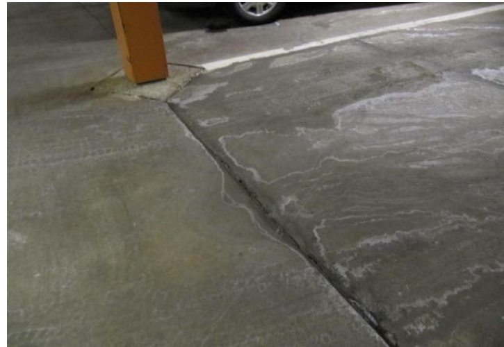
Control joint between parking bay and drive aisle.
