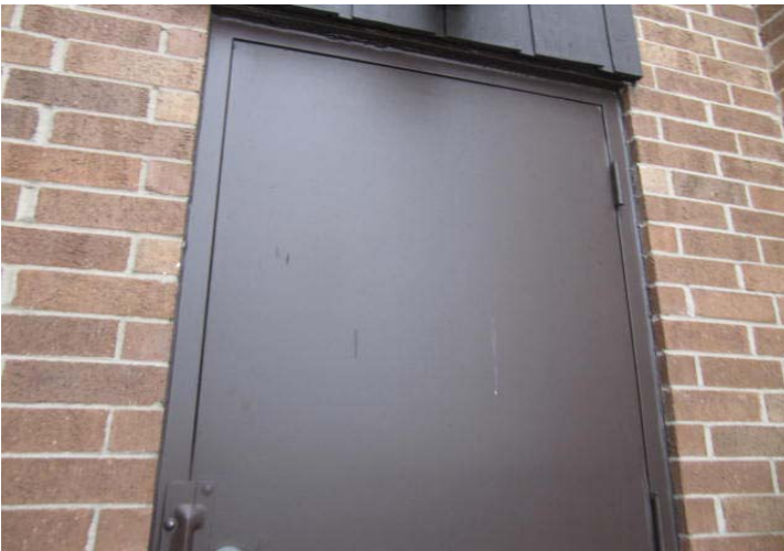
Paint finishes at exterior face of door.
