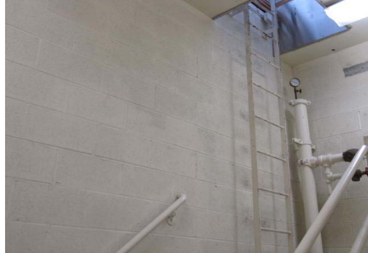
Painted concrete block walls at stairwell.
