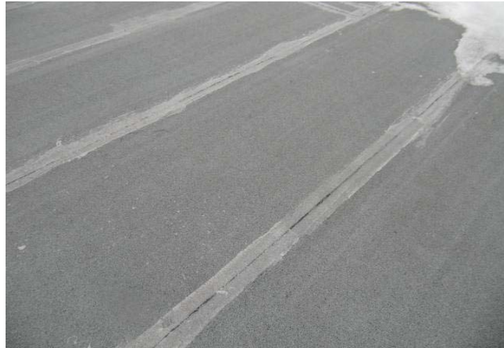
Overview of flat modified bitumen roof.
