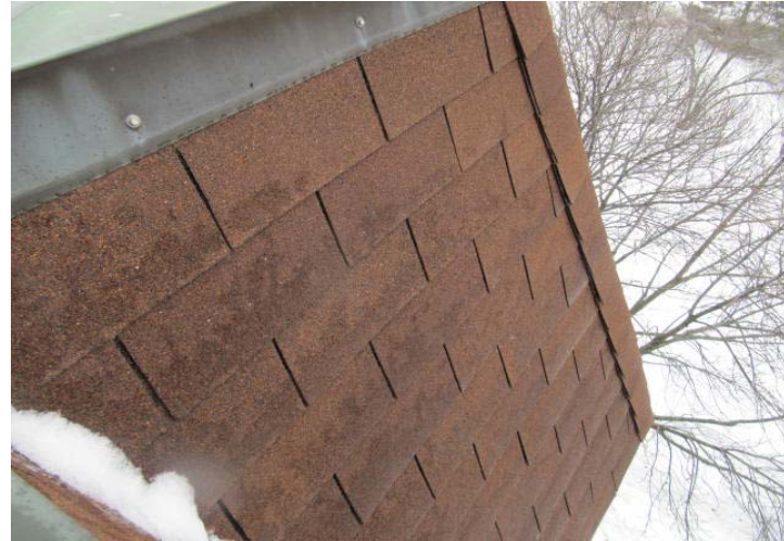
Asphalt shingles, in fair condition.
