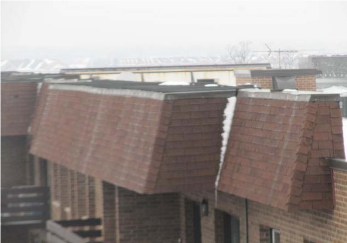
Asphalt shingles at mansard roofs.
