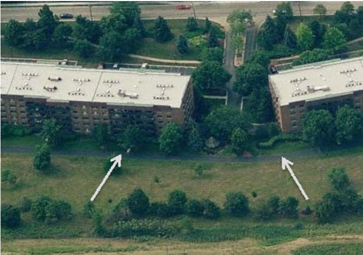
Aerial view of pavement at fire lane.
