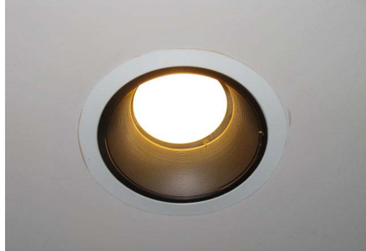
Typical recessed can light.
