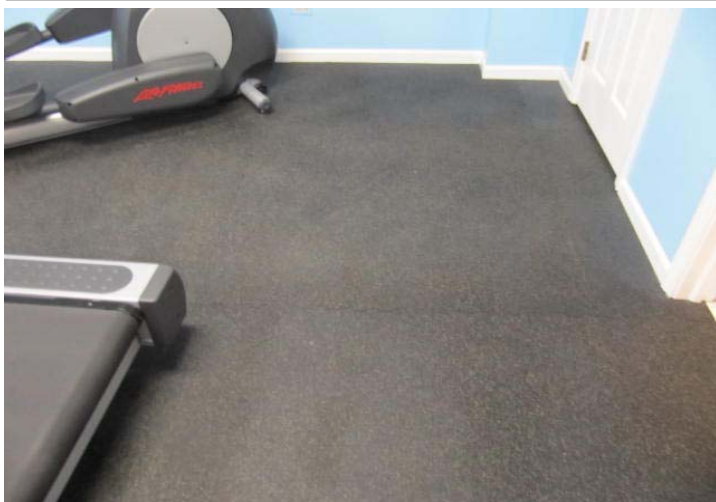
Overview of rubber sports flooring, installed in 2013.
