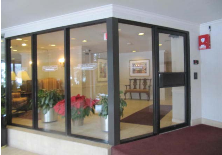
Commercial store-front style glazing with entry door.
