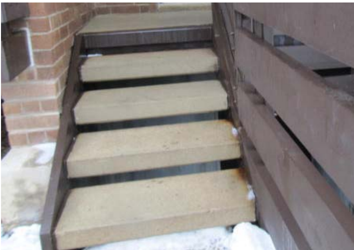
Concrete stair treads leading to private stairwell.
