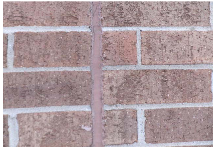
Sealant at building masonry control joint.
