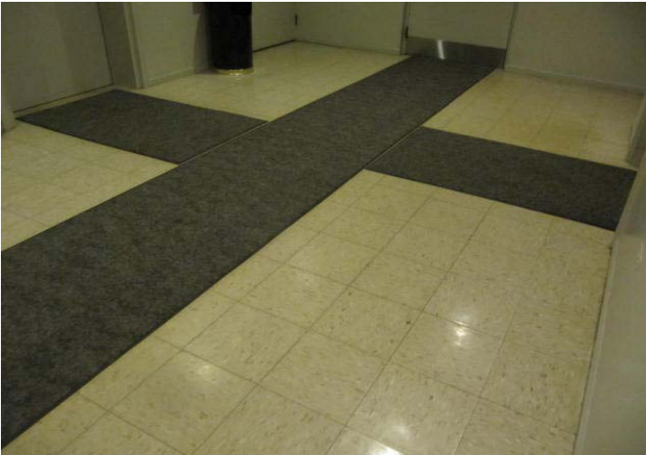
Overview of vinyl tile at lower level (with floor mats).
