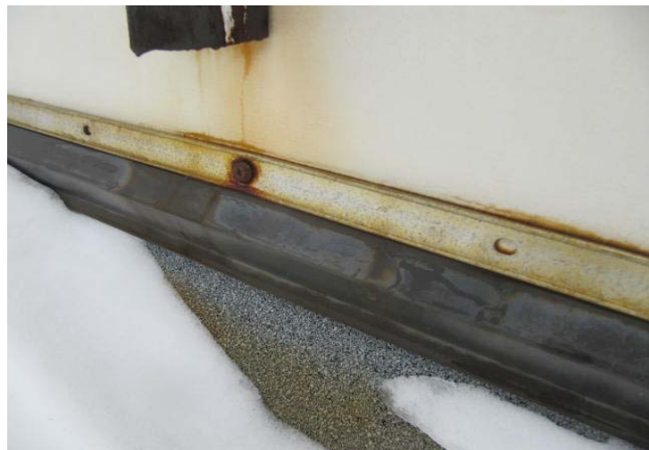
Transition / flashing between flat roof and parapet wall.
