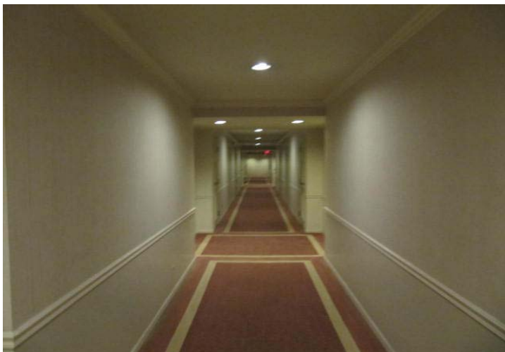
Overview of painted walls and ceiling at hallway.
