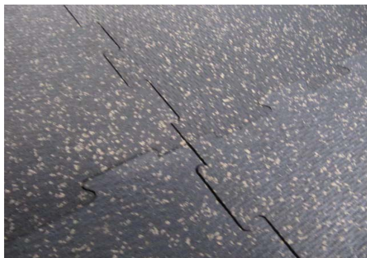
Interlocking floor tiles, in very good condition.
