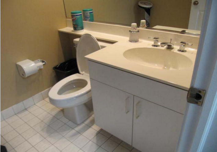
Overview of bathroom at exercise room.
