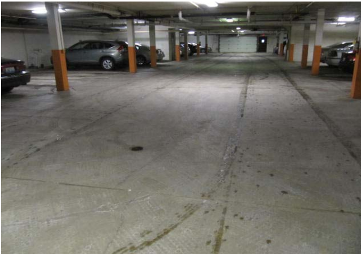
Overview of concrete garage floor.
