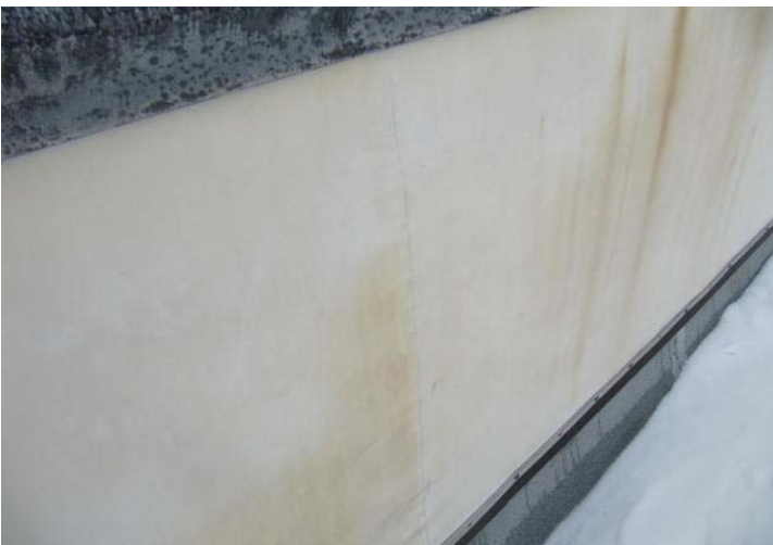
TPO membrane at vertical parapet wall surface.
