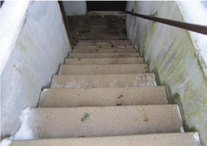
Overview of concrete stairs leading to lower level.
