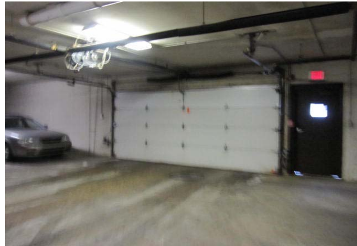
Interior view of garage door.
