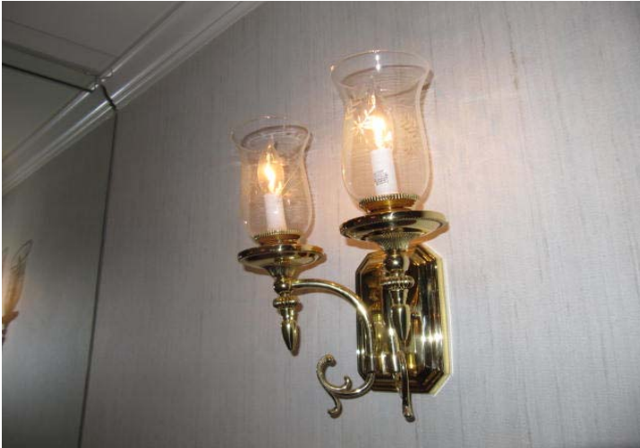
Sconce fixture at entrance lobby.
