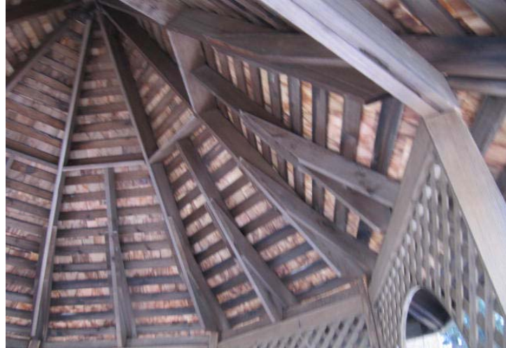
Gazebo roof, replaced in 2013.
