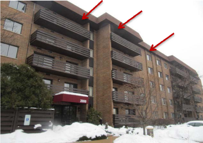
Overview of soffits at mansard roofs.
