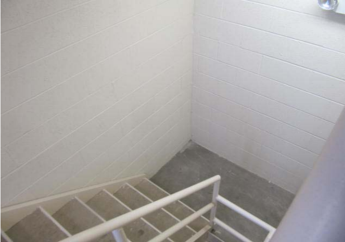
Painted walls at stairwell interior.
