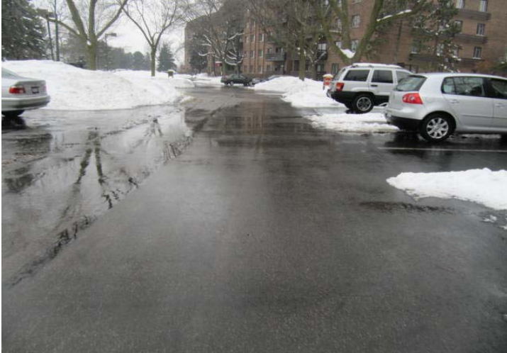
Overview of asphalt pavement at parking lot.
