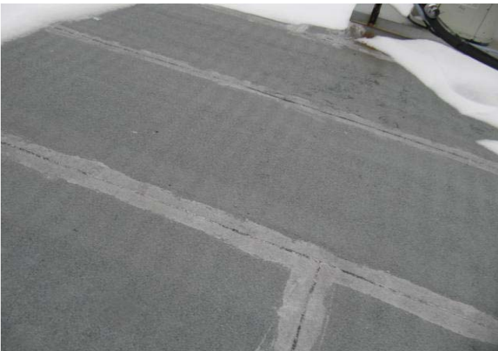
Modified bitumen roof, in good overall condition.
