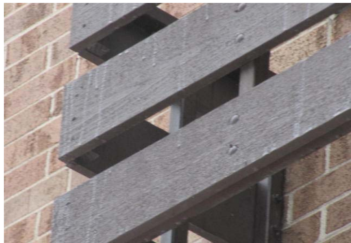
Wood rails and finishes are in very good condition.
