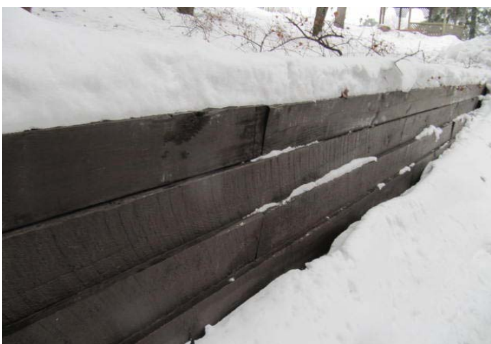
Painted timber retaining wall.
