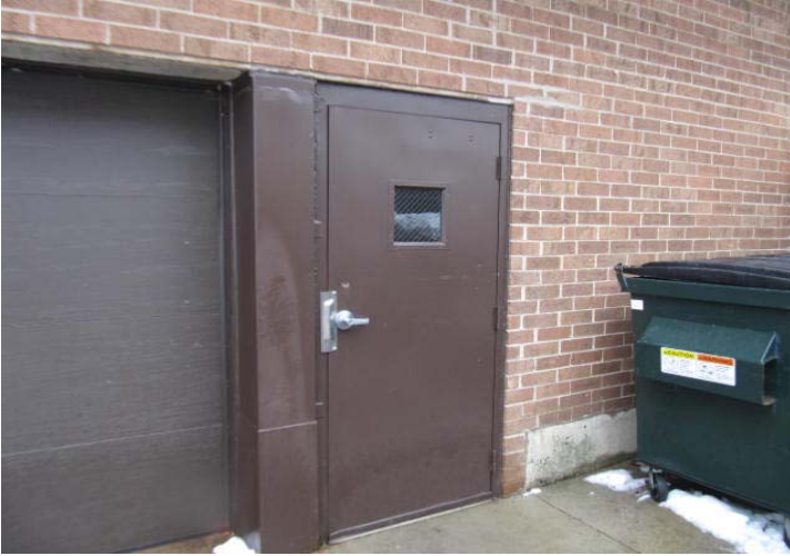
Pedestrian door near garage door.
