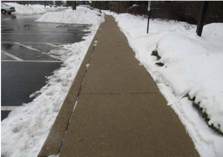
Overview of concrete sidewalk.
