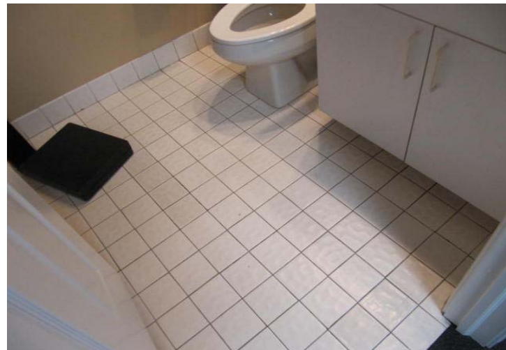
Tile flooring at bathroom floor.
