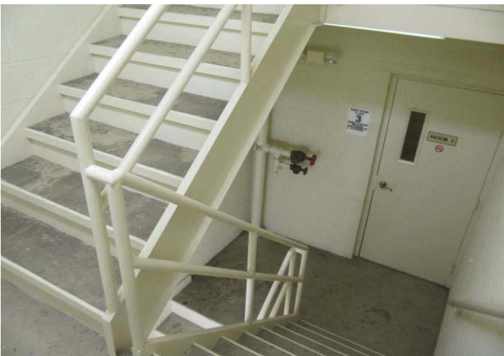
Painted metal railings and stairs.
