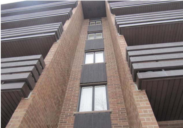
Overview of wood siding between stairwell windows.
