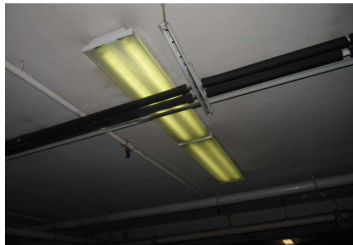
Garage light fixtures are in good overall condition.
