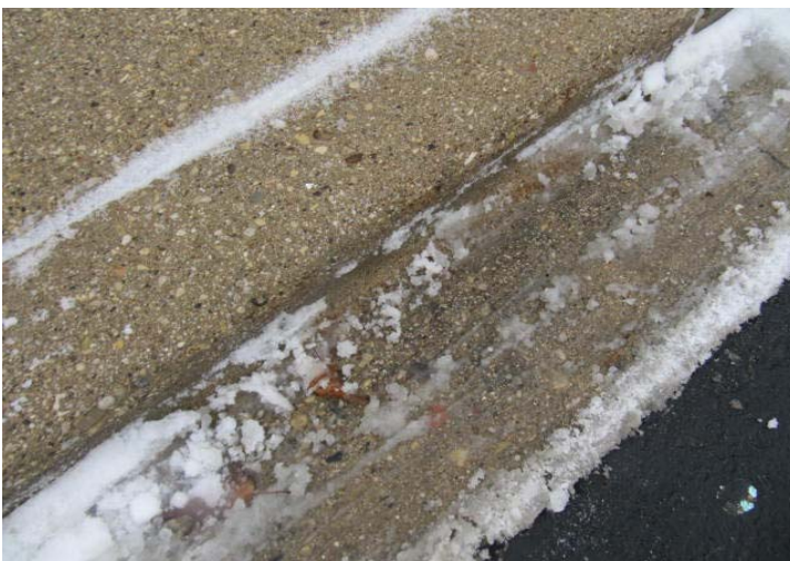
Raised concrete curb and gutter at parking lot.
