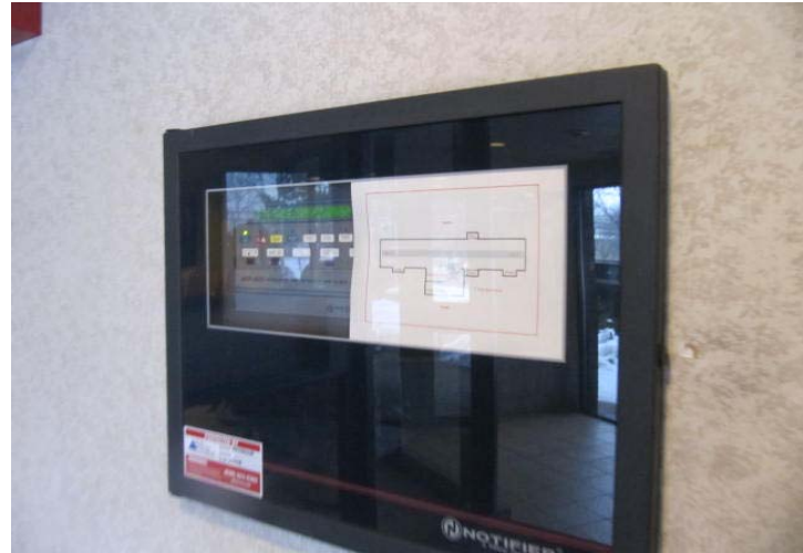
NOTIFIER brand fire control panel.
