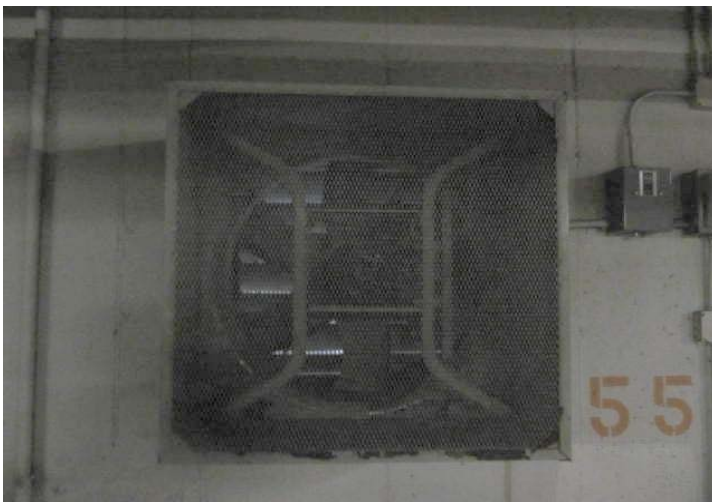
Original exhaust fan, at 30 years of age.
