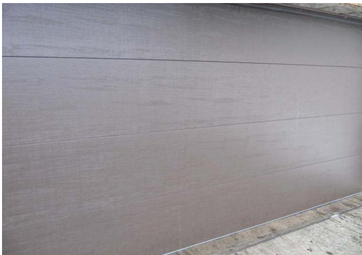
Exterior door finishes are in good condition.
