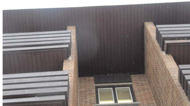
Aluminum soffits, in good overall condition.
