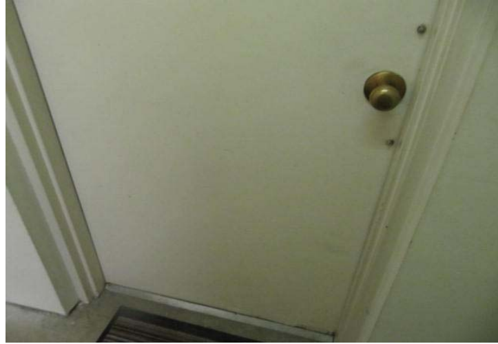
Interior view of door at private stairwell.
