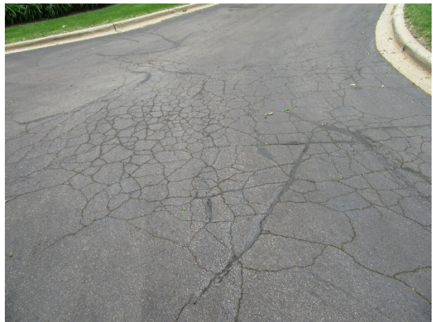
Alligator cracks
