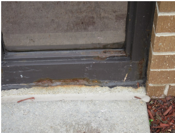
Frame deterioration
