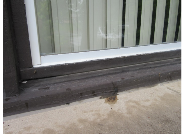
Frame deterioration
