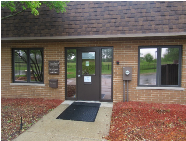
Windows and door
