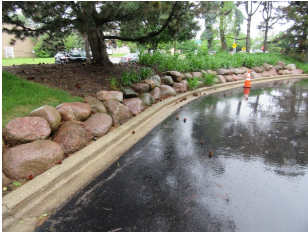
Stone retaining wall
