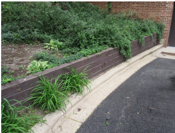
Retaining wall overview
