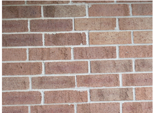
Masonry crack
