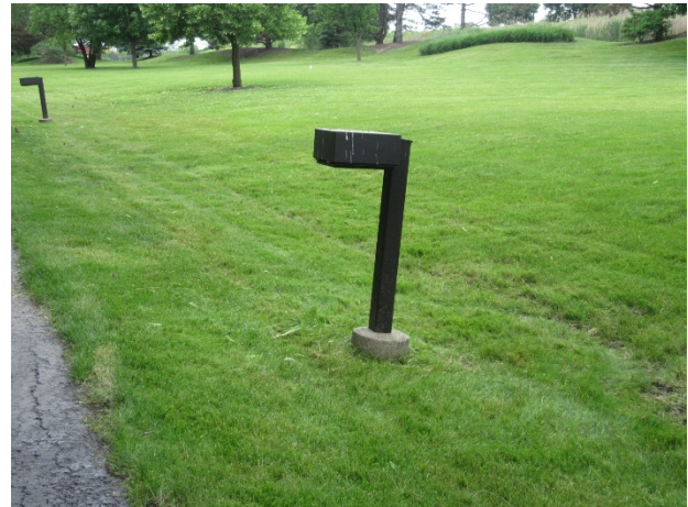
Light pole lean
