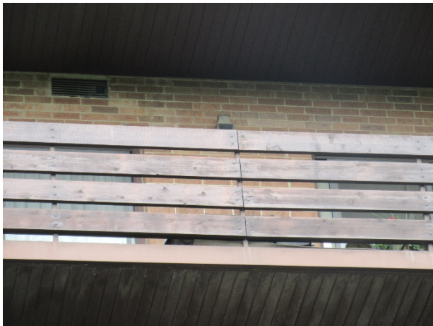
Finish deterioration
