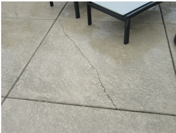
Deck crack
