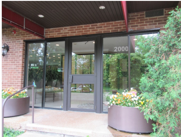
Entrance door and windows
