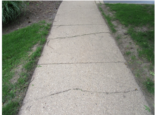
Sidewalk cracks
