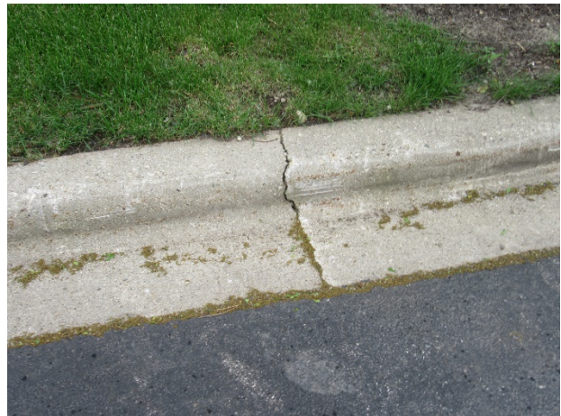
Curb crack
