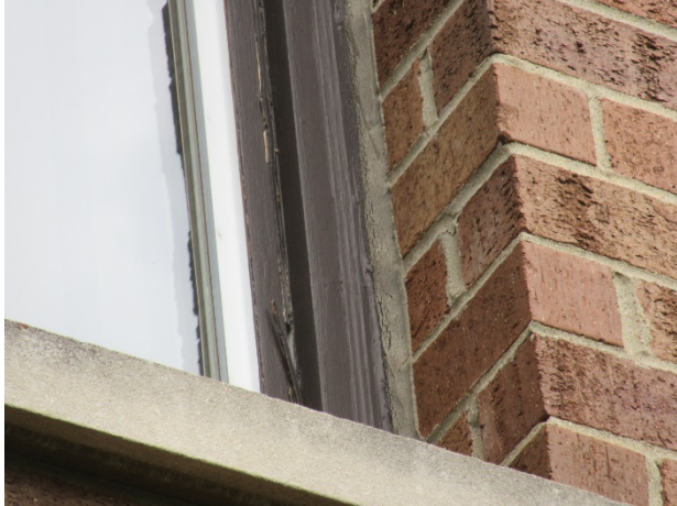
Sealant deterioration
