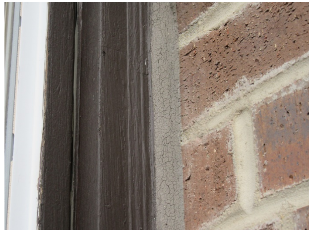
Sealant deterioration
