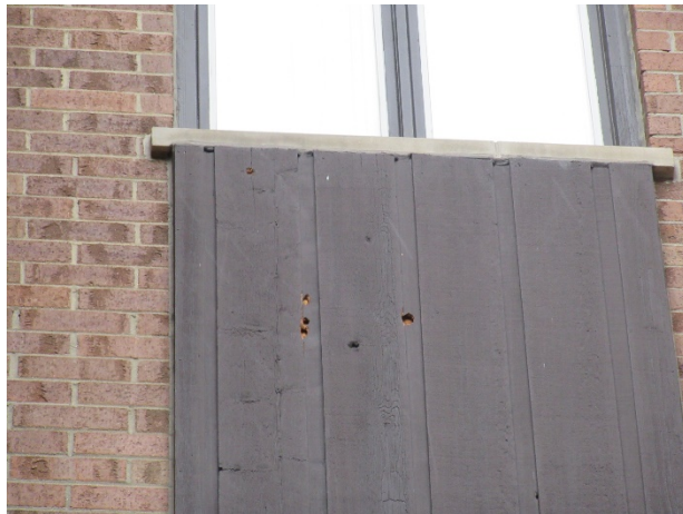
Siding damage
