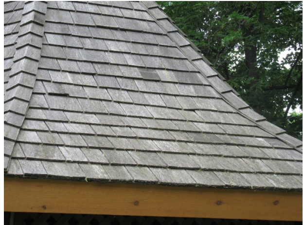
Shingle lift and split
