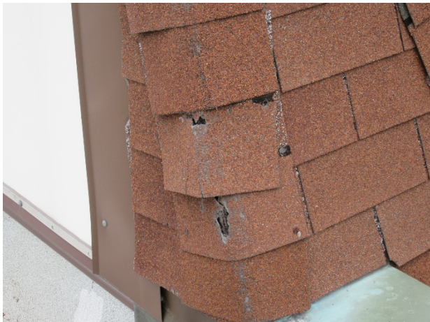
Shingle damage
