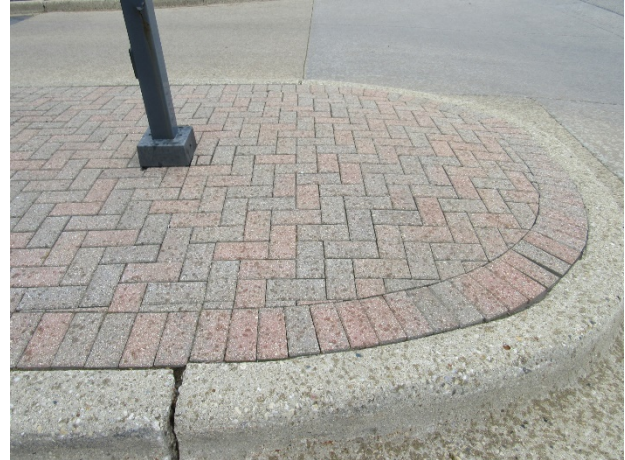
Pavers in good condition
