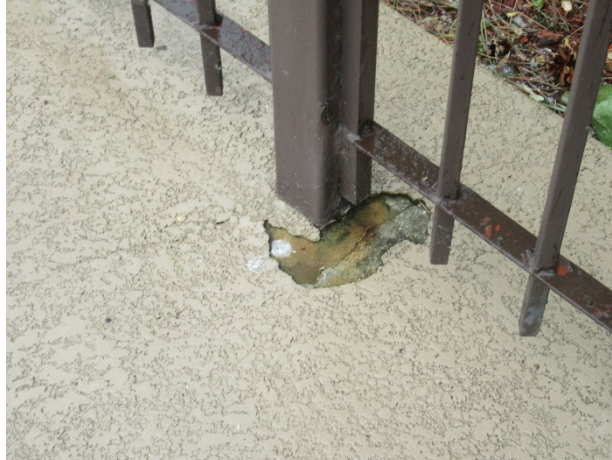
Coating deterioration
