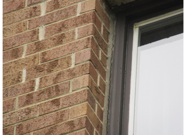
Adhesion failure
