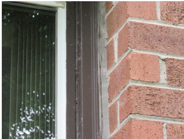
Cohesive failure
