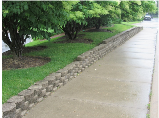
Masonry retaining wall at west end of property
