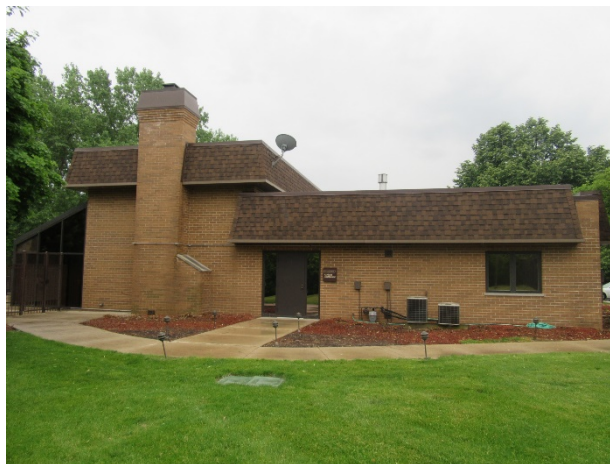
Mansard roof overview
