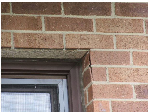
Delamination
