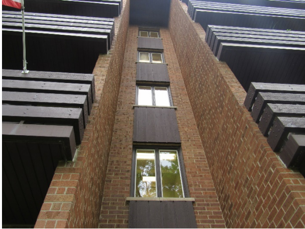
Common windows at private stairwells
