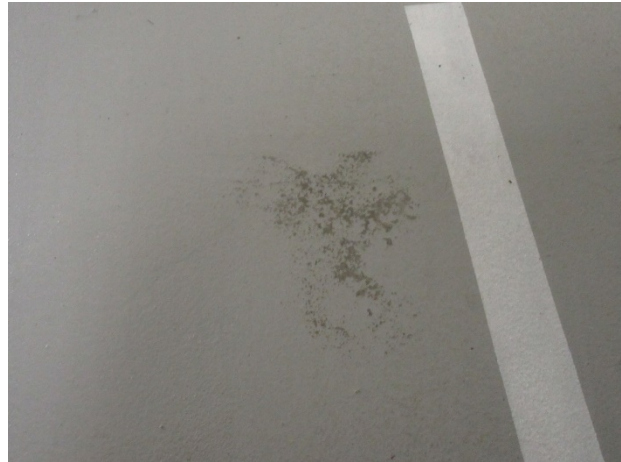
Finish deterioration
