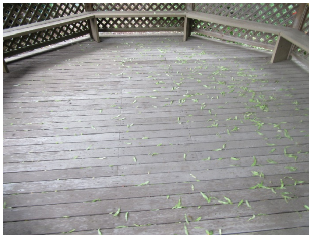
Deck board overview
