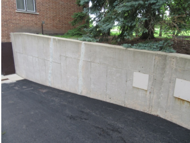
Concrete retaining wall at east end of 2000 building
