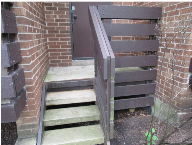
Metal pan staircase and landing
